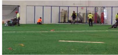
both of its 190 by 85 feet indoor fields received new two-inch high artificial turf. The original turf was long overdue for replacement.
